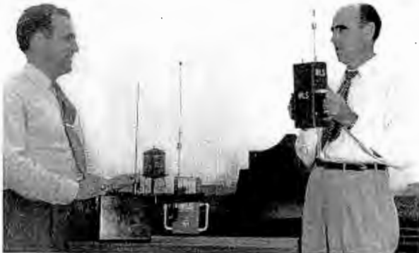
ROY HUBERTY and Vern Fulton test short wave remote transmitter and receiver equipment on the roof.
