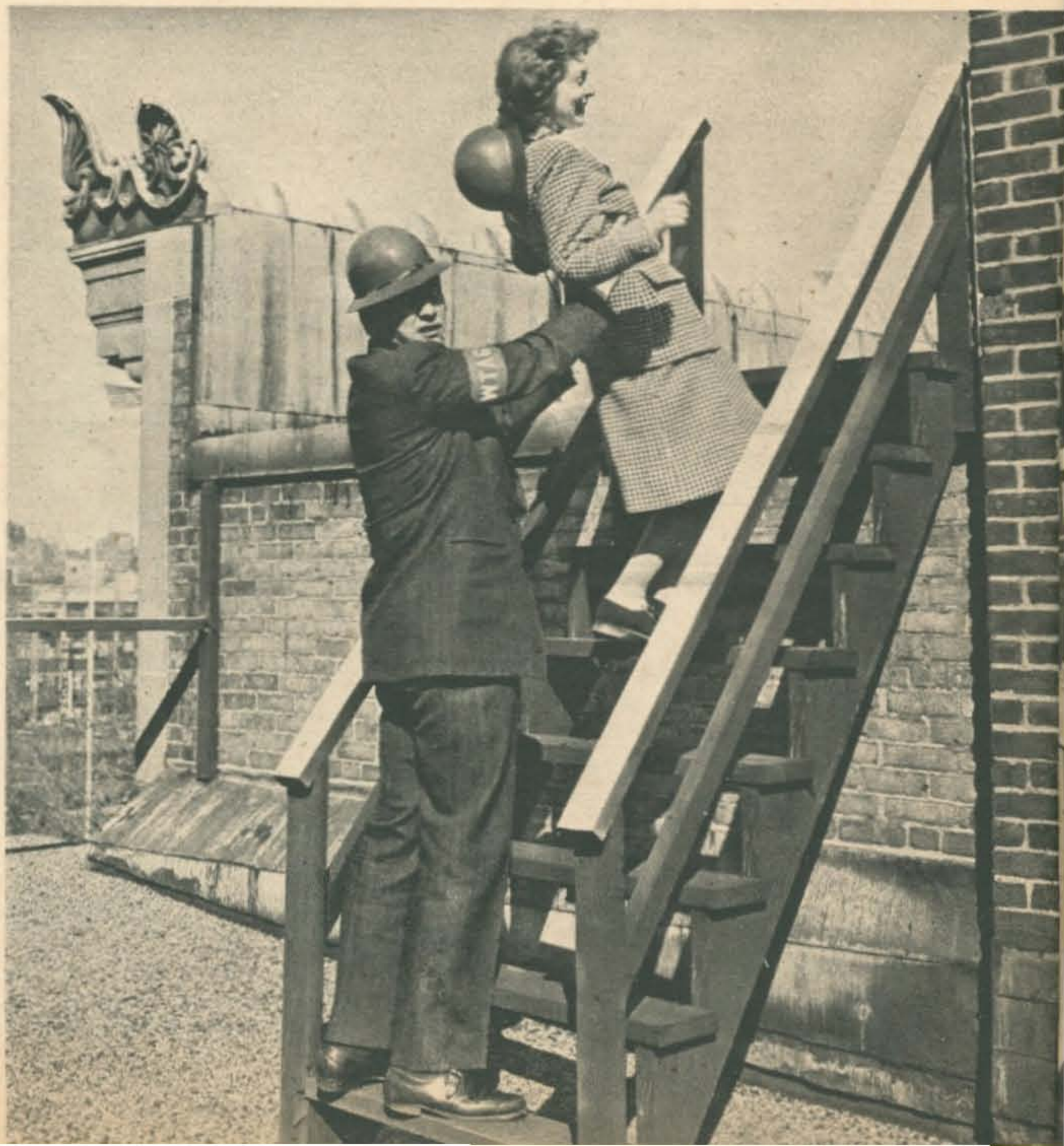
ONE OF THE STAIRWAYS WHICH CONNECTS VARYING ROOF LEVELS IN THE DEFENSE AREA.
