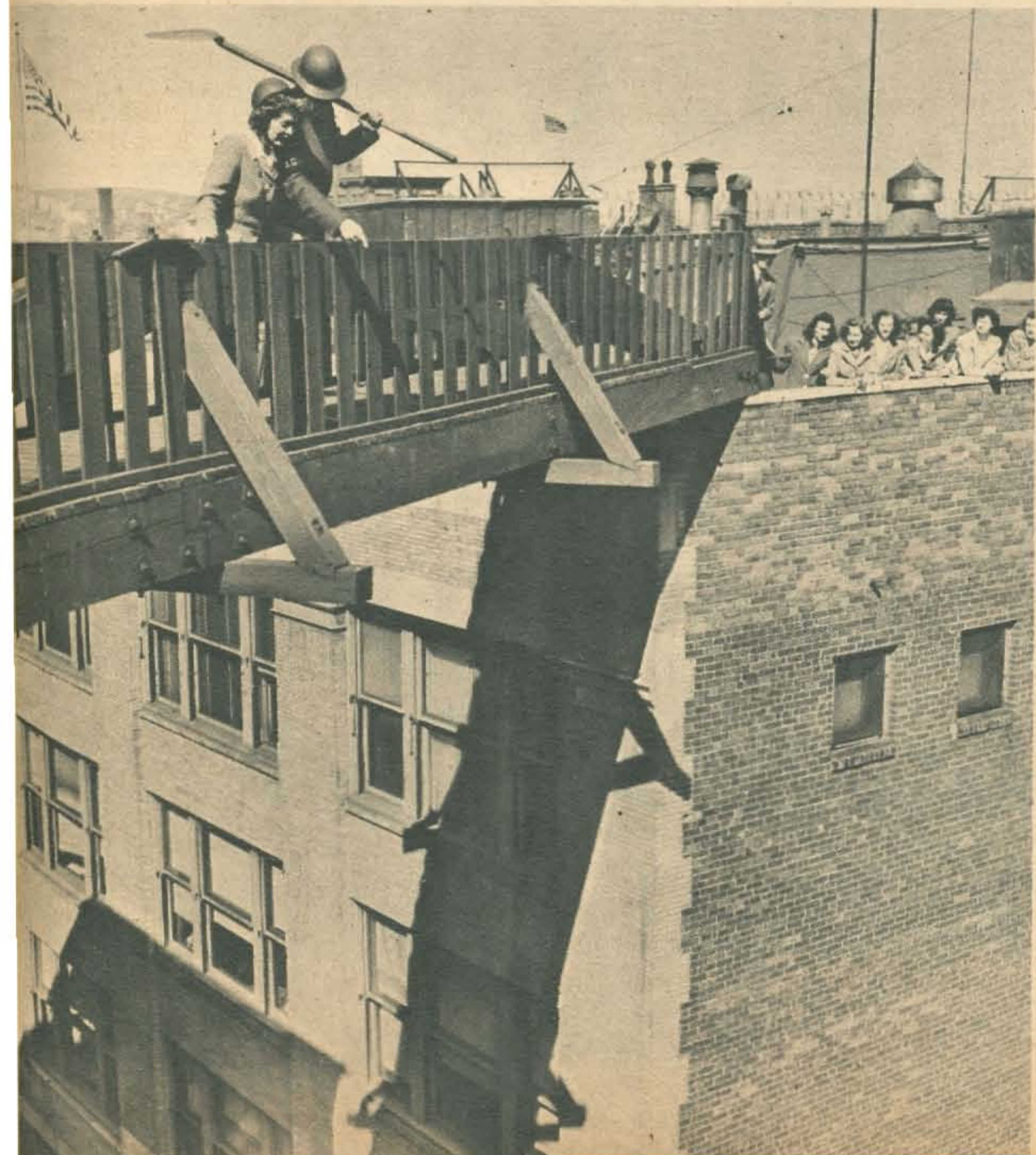
A 7,000 LB. CONNECTING BRIDGE JOINS WTAG'S BUILDING WITH ONE ACROSS THE STREET.
