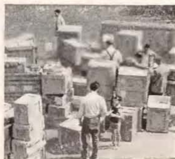
Part of the 401 cases of RCA equipment shipped to Berlin for television demonstrations.
