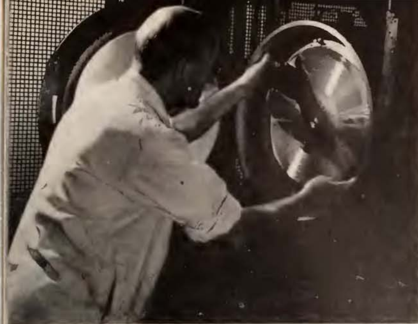
9 - gold sputtering is a must if transcriptions are to be of top quality. Recording is sputtered right after being made
