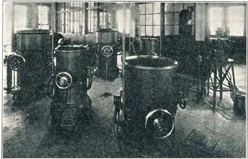
The six arc-convertors of the San Francisco terminal.
