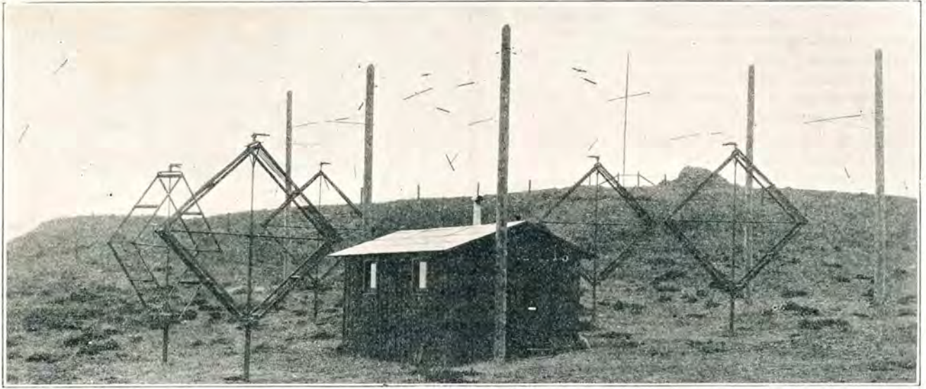
Daly City receiving station. The five loops, and another loop not shown, are connected to six receiving sets inside, from which the head telephone leads are extended through buried conduit to the city offices far below.
