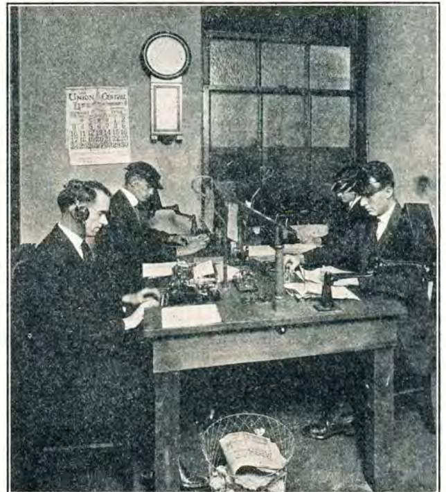
All these boys in the city office have to do is to see how fast they can telegraph. Two are sending and two receiving. There is a table like this for every two arcs.
