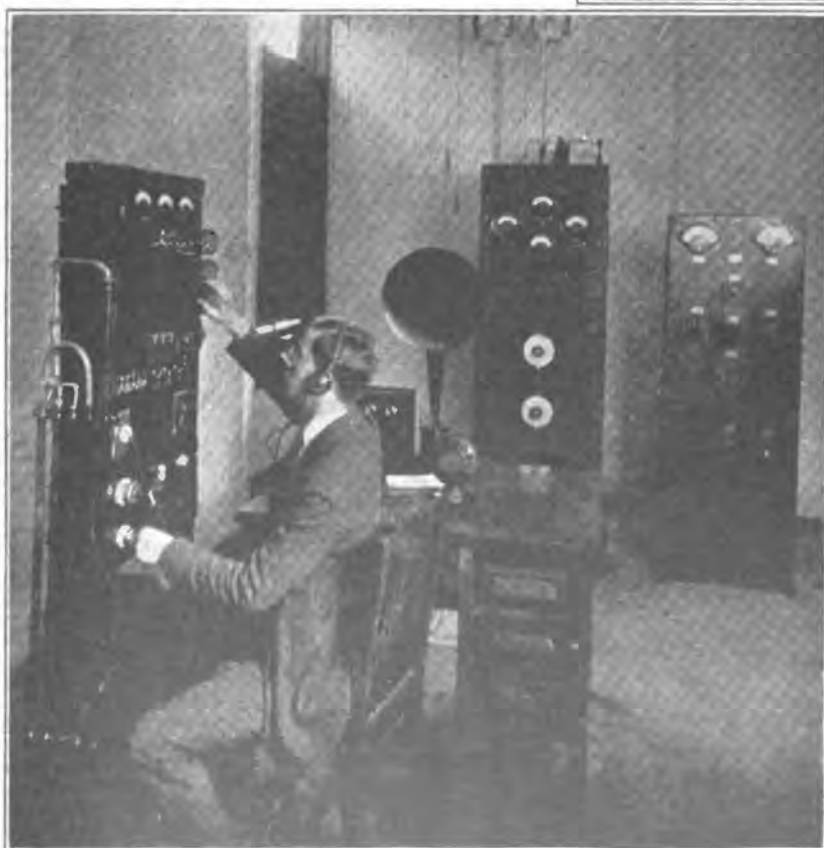
500 Watt Western Electric Radio Telephone Equipment in the Wanamaker Broadcasting Station at Philadelphia, Pa., by Means of Which Music From the Wanamaker Grand Organ Has Been Heard at Berkeley, Calif., and San Juan, Porto Rico.
