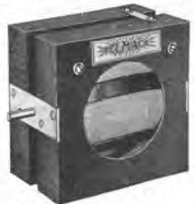
Fig. 38. Unmounted Variometer.
