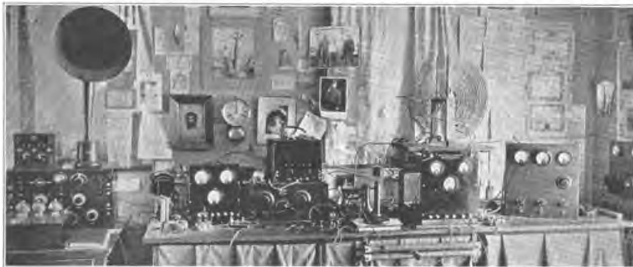
Radio 6XAD, Avalon, Catalina Island, California. Kennedy Long Wave Receiver, Grebe 2-Step Amplifier and Western Electric Loud Speaker at Left. On the Main Operating Table are ICW Transmitter Using Two 50-Watt Tubes Radiating 6.1 Amp. on 240 meters, Grebe CRS with Special Western Electric 2-Step Amplifier, CW Transmitter Using Four 50 Watt Tubes Radiating 7 Amp. on 370 Meters, and ICW Transmitter with Four 5 Watt Tubes Radiating 2.9 Amp. or 220 Meters. At the Right is a Motor-Generator Set Delivering 1500 Volts dc to 200 Watt Transmitter.
