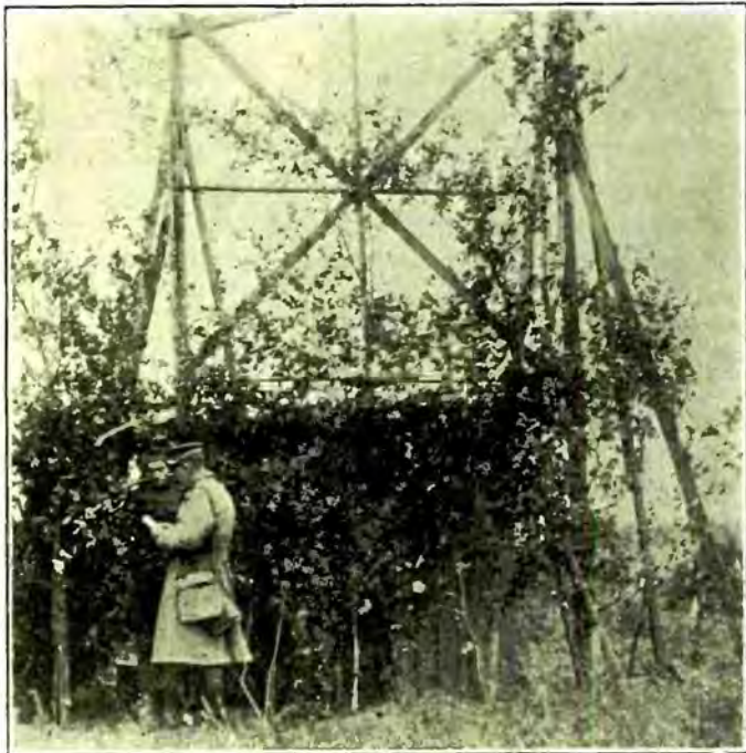
American Direction Finder Near Front Lines Day Previous to St. Mihiel Attack by American Troops. These Stations Were Located About Five Miles in Rear Front Lines and Twelve Miles Apart. The Hut and Loop Are Camouflaged in Order That the German Aviators Cannot Locate the Station. Loop Used is Ten Feet Square.
