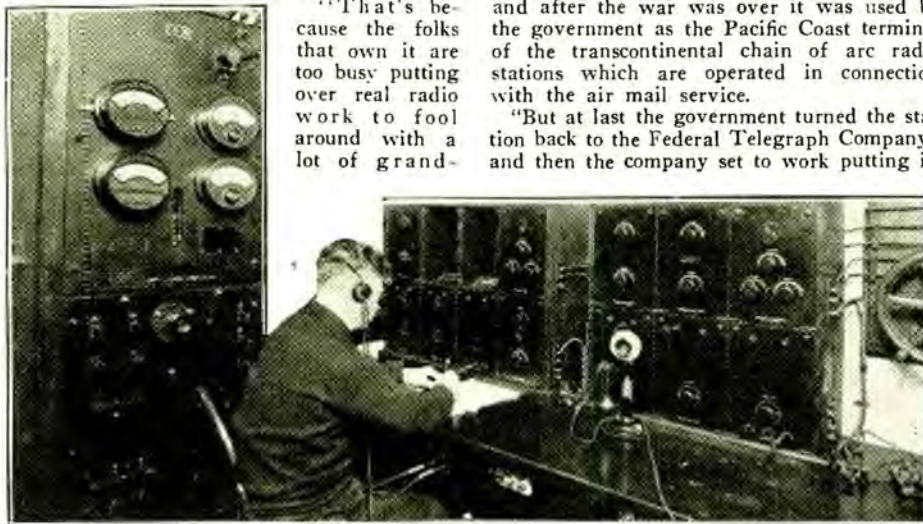
Receiving-room. From left to right, arc-control panel, 1,700-3,000 meter CW receiver, and 600-meter spark receiver. The operator hears simultaneously 600-meter spark signals in one telephone receiver and 2,400-meter CW in the other.
