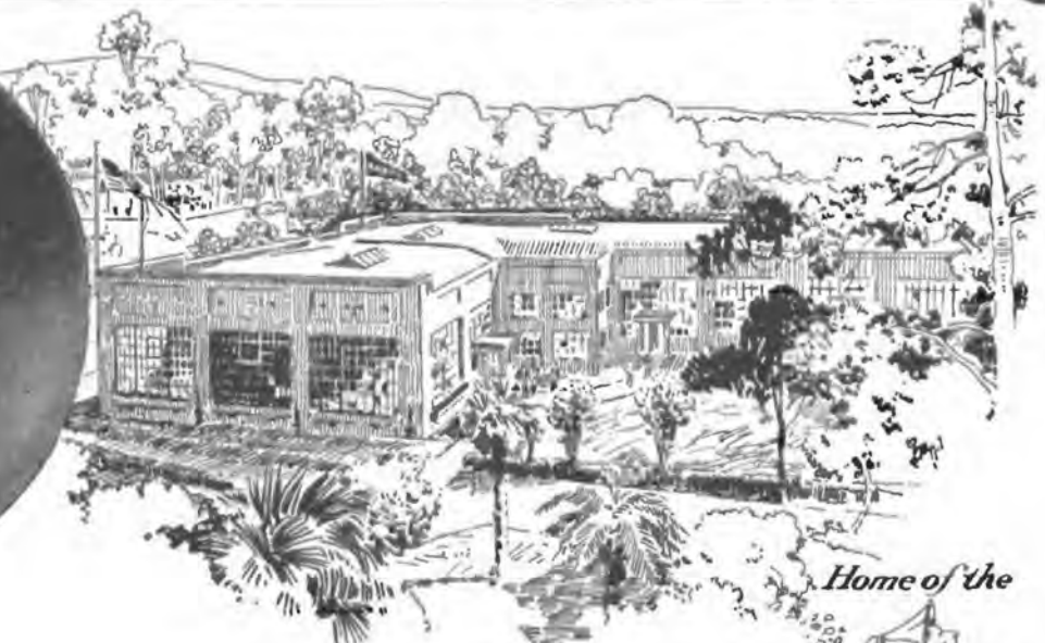
The Plant of the Magnavox Co., Oakland, California—one of the show factories of the Pacific Coast.
