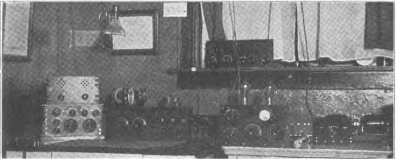
Interior of Station at 9DVA
