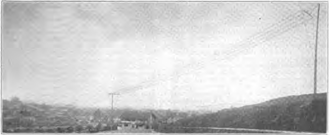
View of Radio Masts and Antenna at KZY
