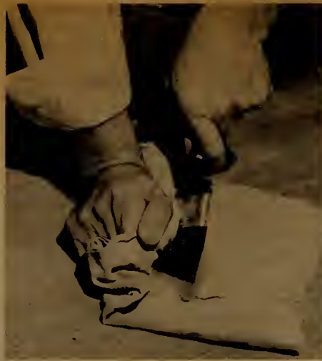
3. Cotton cloth for wiping should finally show no paint stains, and the brush should be dry as possible.
