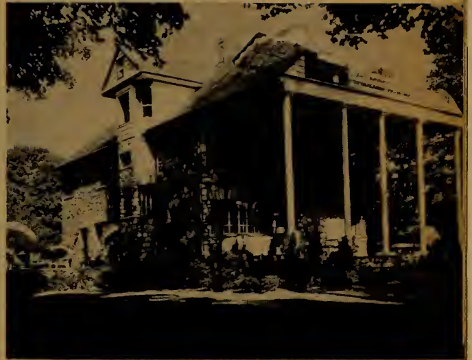
AFTER: Two years later, with Georgian columns, stone walls, landscaping, it is hard to believe it's the same place.
