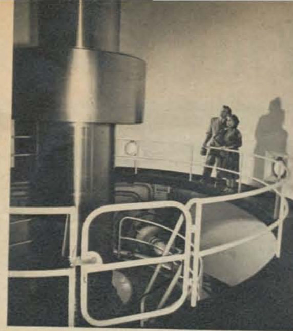
At Grand Coulee dam: awesome machinery . . .
