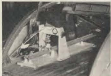
The "long-lines" type 5 meter transmitter installed in an amateur's car. These sets did trojan service in "short haul" communications.
