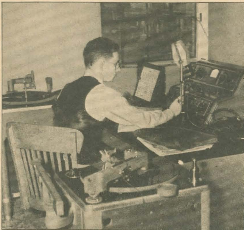
WBOE sends "master lessons" to 115 Cleveland schools. J. D. Woodworth, technical director of public-owned station, is shown at controls
