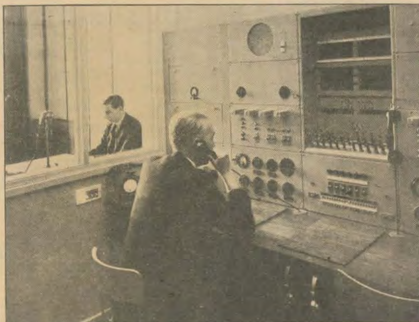
Listeners to HBH (18.48), Switzerland, may hear League of Nations broadcast Sunday morning at 10:45 a.m. EST. Above: View of the recently finished control-room in the League of Nations Palace
