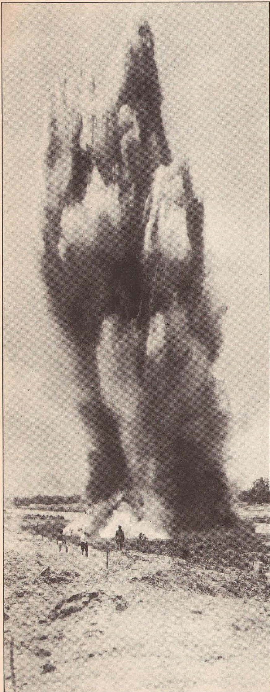
One of the most interesting jobs ever done by dynamite has been the use of it in many parts of the country to make new courses for streams. Above is a dynamite blast which built a new channel for a stream in Mississippi
