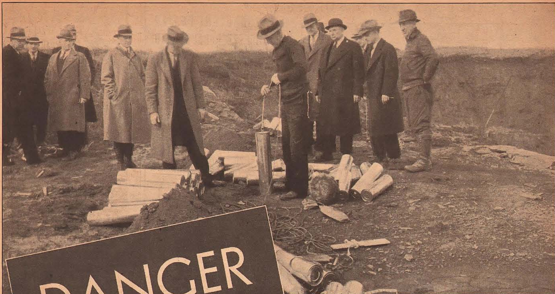
Authority on large dynamite blasts, Samuel Russell will tell all on "Americans At Work" Thursday. Above: Russell placing charges of nitramon preparatory to a shot at quarries of cement company in Pennsylvania
