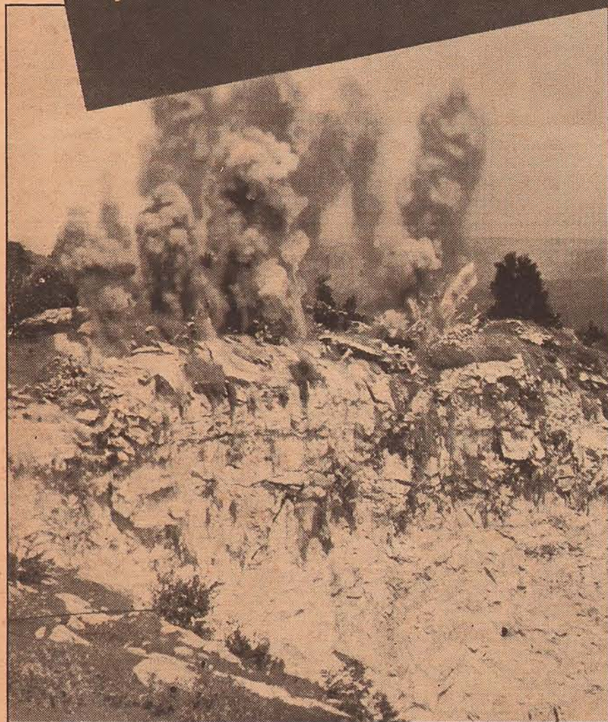
In some quarries dynamite shots are used to bring down the stone. Tunnels are driven into the side of a hill and dynamite is placed in the tunnels. This picture shows such a tunnel-shot as dynamite explodes
