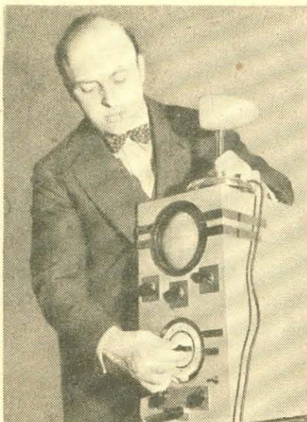
The resonoscope tests pitch, can also be used with great accuracy for tuning all kinds of musical instruments
