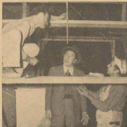
While new CBS-KNX building was under construction, Comedian Joe Penner, who will be among those using it, looked on
