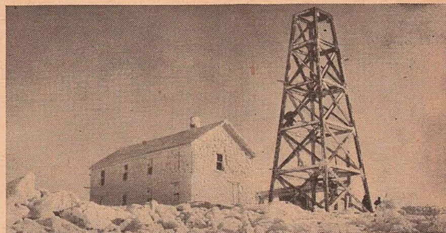
On Feb. 20, the Yankee Network inaugurated the country's most complete radio weather forecasting service. Construction of the observatory (above) on Mount Washington was halted many times because of snow, high winds
