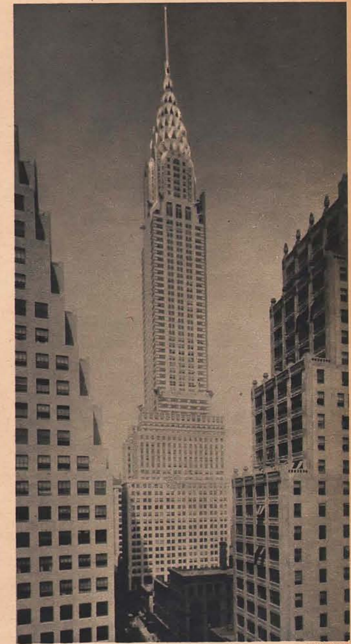
33 CBS transmitter is in new studios atop the Chrysler Building in New York. Success of this new form of entertainment depends on a long but fruitful trial-by-error
