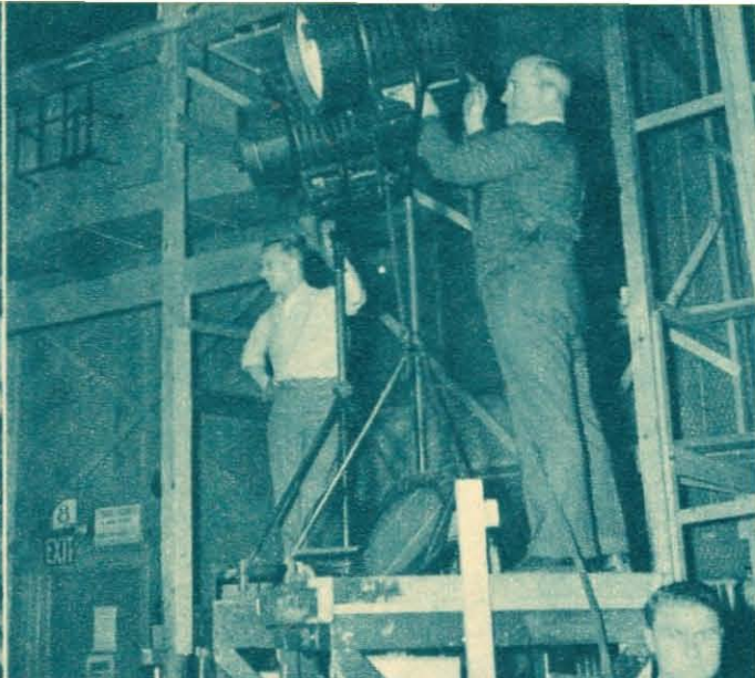
Powerful Kleig lights on movable platforms make special light-effects possible. Sometimes as much as 10,000 watts are used to light one set of a movie short such as this
