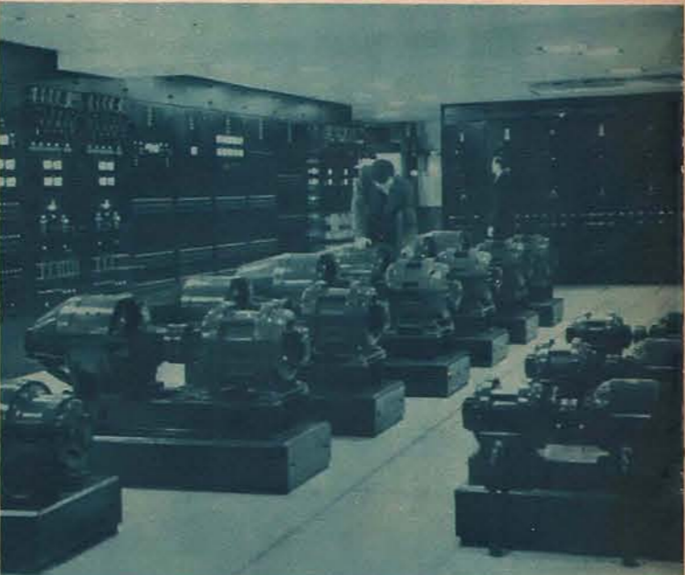
4 Motor generators (above) develop the power used. Stored in batteries to assure a smooth, uniform flow, the reserve could run Radio City for 72 hours!
