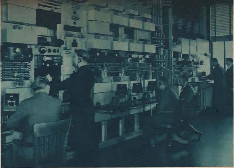
8 Wires, such as those to the right, carry broadcasts over the nation. But because sending signals over wires weakens them, booster stations (above) are needed every 50 miles to amplify them, restore their strength
