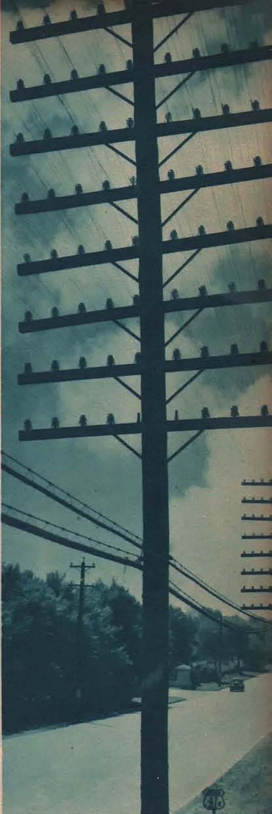
8 Wires, such as those to the right, carry broadcasts over the nation. But because sending signals over wires weakens them, booster stations (above) are needed every 50 miles to amplify them, restore their strength
