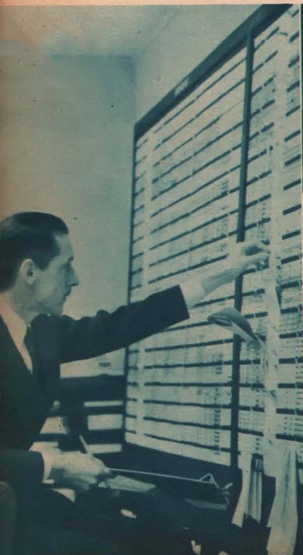
3 A miniature of power lines (above) reveals the location of any power failures. All power equipment is installed in duplicate to cover emergencies
