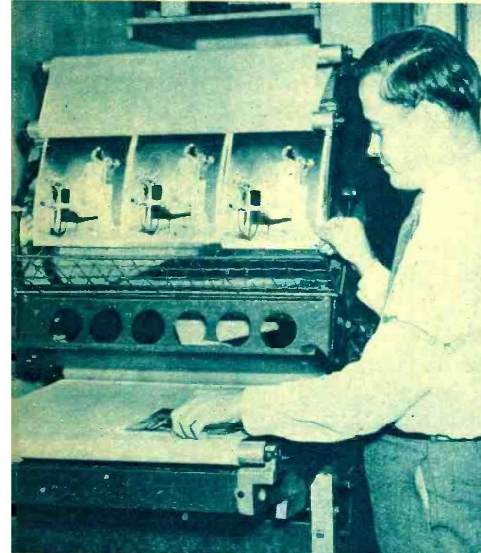
12 After the prints are developed, and "fixed" in hypo, Dick Schroeder dries them on cloth by heat & air in this machine
