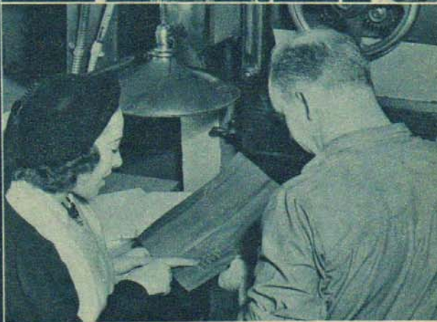
11 The message for the inside of the card is engraved on a brass block, which is used in the engraving machine operated by George Young, Jr. (above). This machine exerts from 4 to 5 tons pressure on the paper!
