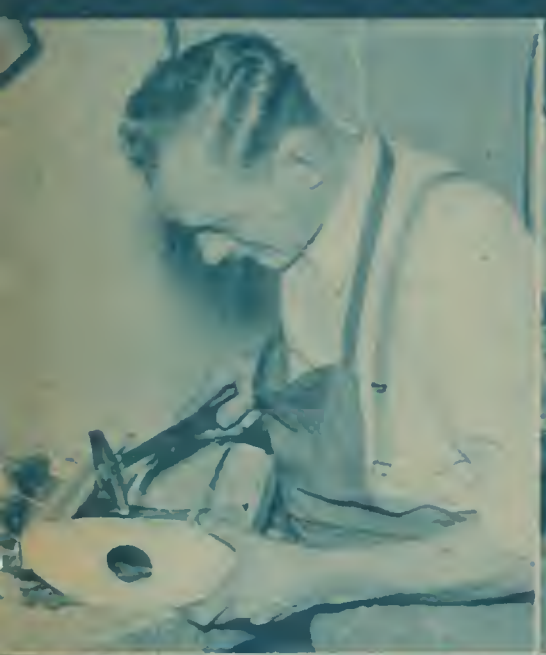
12 Making the body frame. Basswood is used, because it's soft and light, won't check or split
