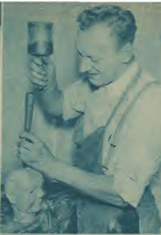
6 Between the two center pieces of wood there is a layer of paper, so that the head can be split without being broken
