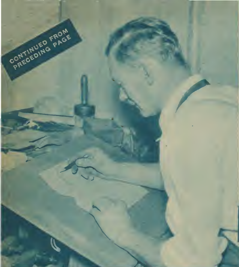
1 Frank Marshall's first step in dummy-making is to draft the head of the dummy on heavy paper. After the profile and portrait have been sketched, they're cut out for patterns
