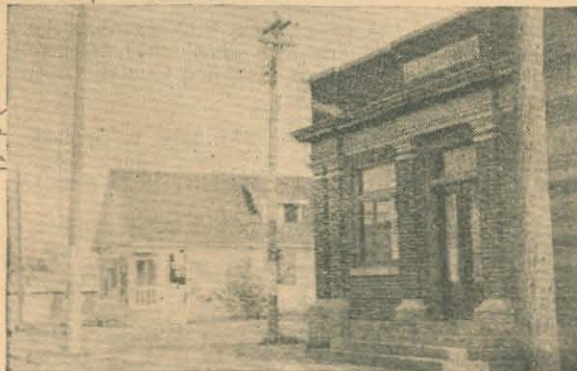
The state bank at Kaleva, Michigan, where the cashier (Mayor of Kaleva) was killed and where the loot was stolen
