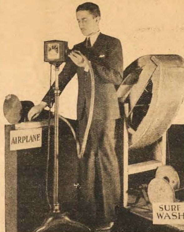
Ray Kelly at work in his sound effects laboratory. Note the canvas container for dried peas, used to create the sound of waves washing upon a shore
