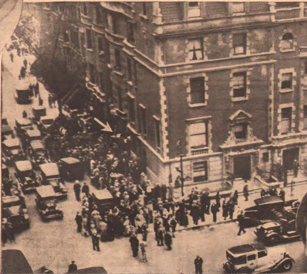
The building at 303 West 90th Street, where Crowley was cornered by a cordon of 800 policemen summoned by short wave radio calls
