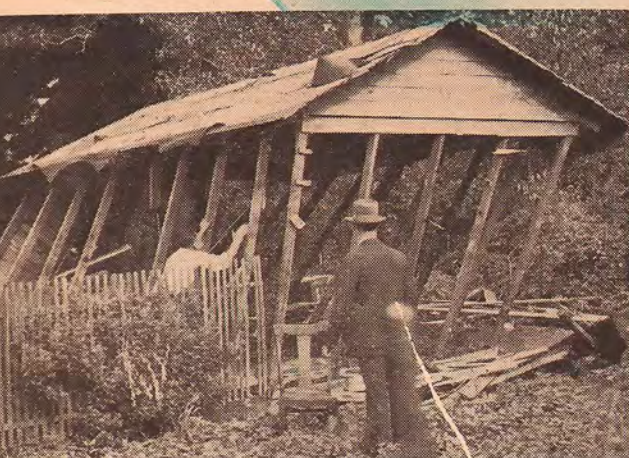
Last stages of demolition of Hauptmann's garage
