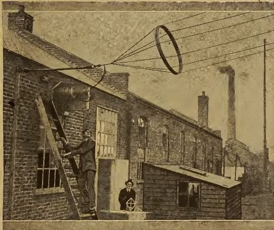
5XX, Chelmsford, England, working on 1,600 meters with a power of 25 kilowatts, was one station enlisted in the recent international tests, November 24 to 30. Although it was, without question, able to outreach practically every British broadcaster, few American fans heard it due to their receiver's inability to reach the wave of 1,600 meters. Picture shows the lead-in at 5XX.
