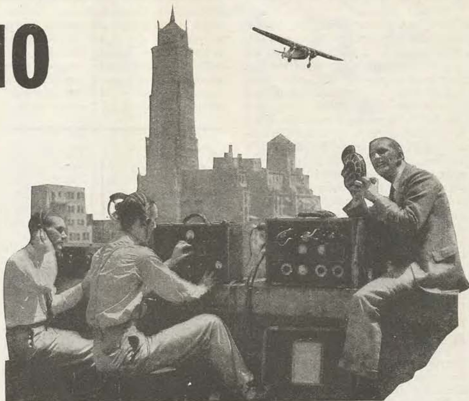
LOOK! HERE'S a thrill! Short wave operation between ground and airplane!
