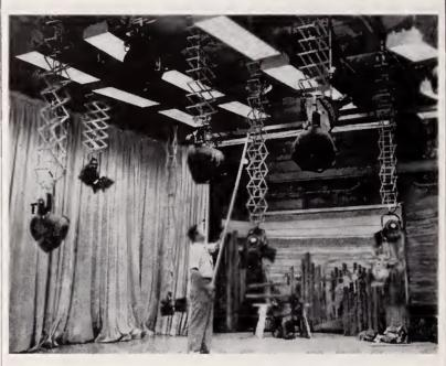
Revolutionary new attachments for all types of TV lights have been installed in the studios of WCAU-TV, Philadelphia. The "skyhook" lights enable engineers to secure many lighting effects which previously required much testing and pre-setting. Lights are attached to overhead power rails and may be suspended or angulated in any direction, plus moved to any direction on the power rails. One man can set the studio lighting in a matter of a minute or two.
