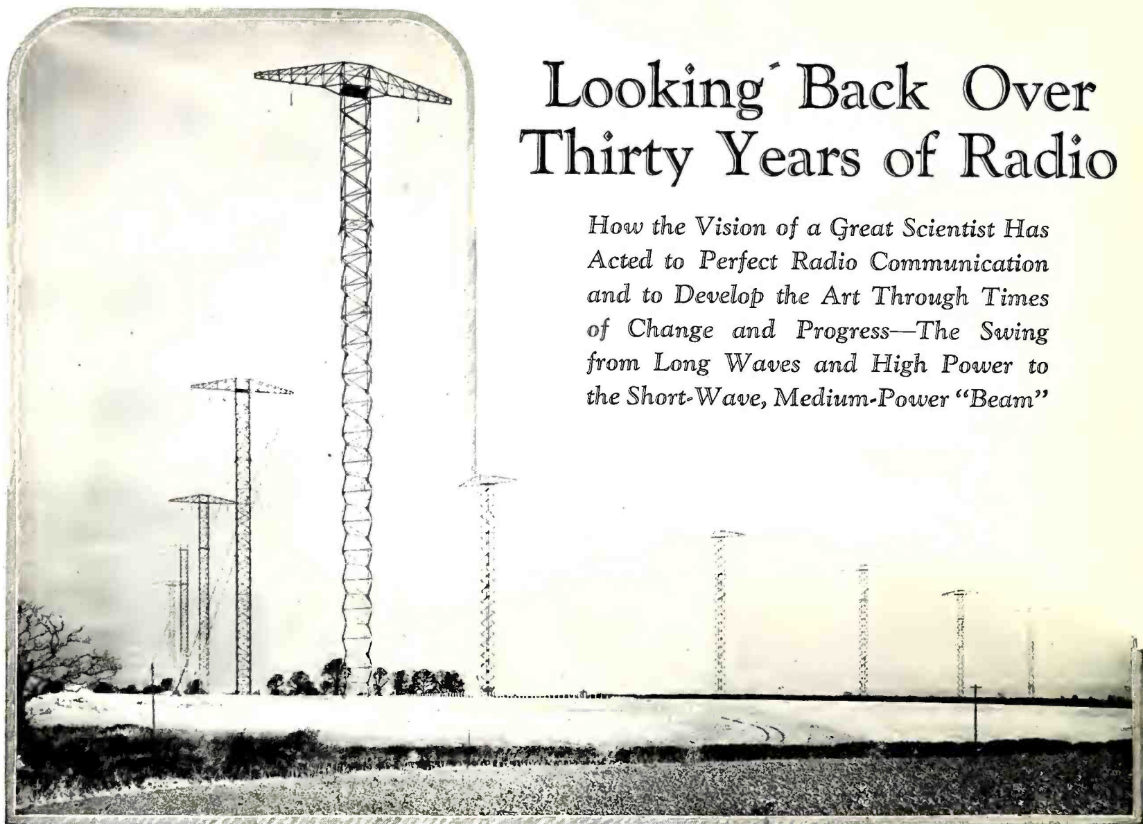
AT THE BRIDGWATER, ENGLAND, "SISTEMA A FASCIO" STATION "Sistema a Fascio," as some are well aware, being the Italian for "Beam System." The five masts to the left are for reception from Canada, while the five to the right are for receiving signals from South Africa
