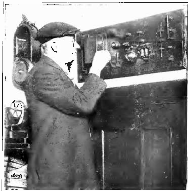
RADIO PRINCIPLES AT WORK IN THE POWER HOUSE The so-called "storm detector" used in the power house of the Brooklyn Edison Company at Gold Street. The principle of the device is merely a simple application of the detection of static charges, which is ingeniously employed to ring a bell. With a warning of approaching storms, the power companies can prepare for the increased load that the darkness will cause
