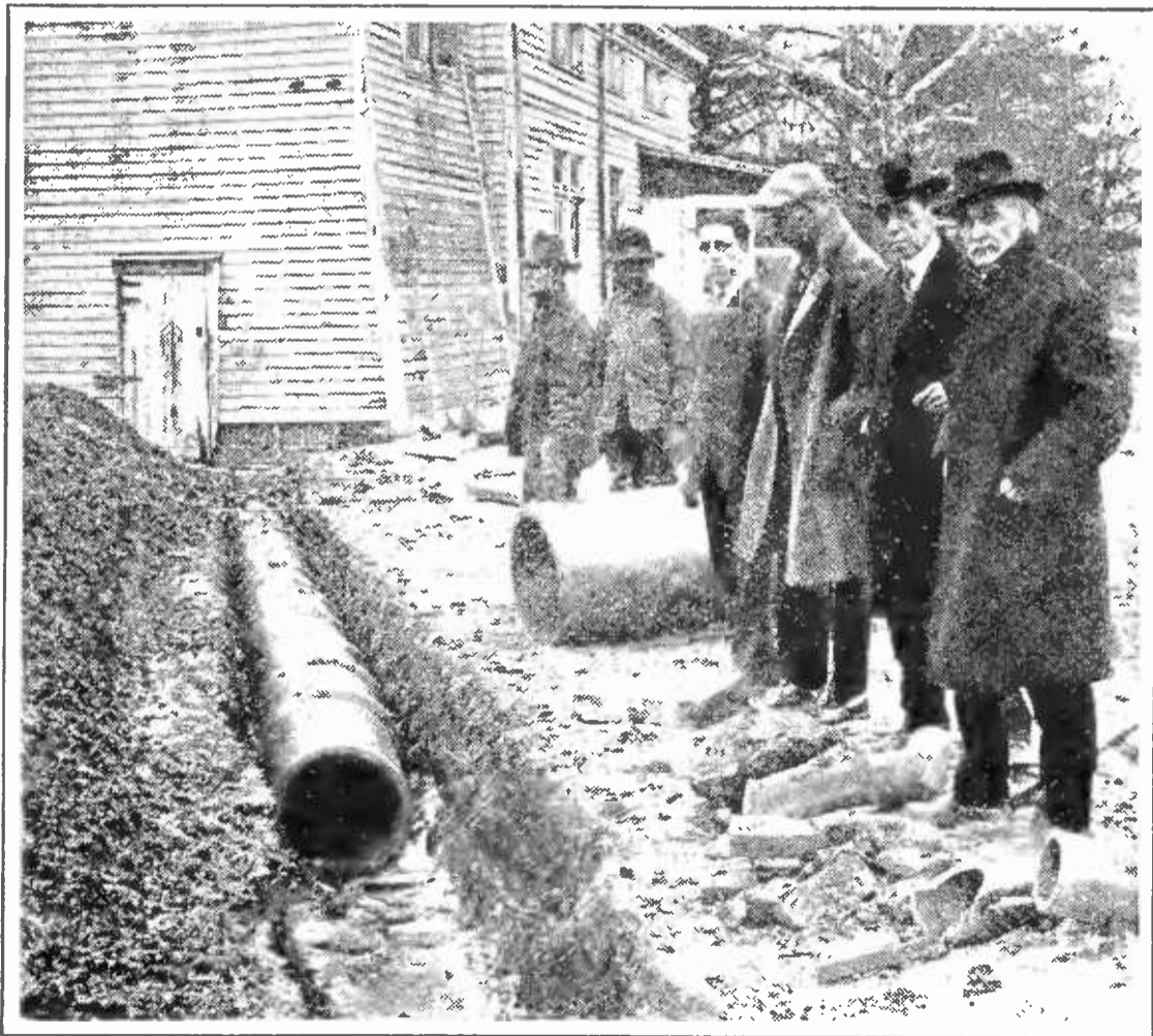
LAYING A ROGERS UNDERGROUND ANTENNA
