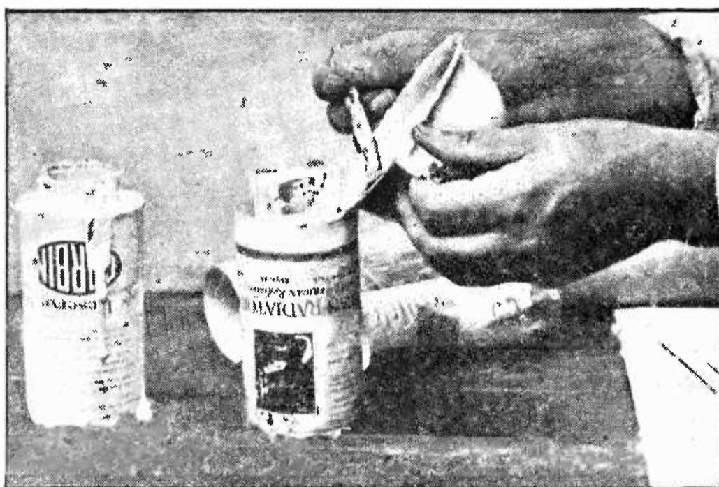
FIG. 5 Molding the porous cup
