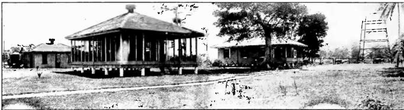
THE RADIO STATION AT TELA, HONDURAS
