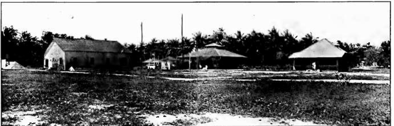
THE RADIO STATION AT SANTA MARTA, COLOMBIA Showing the power house, operating house, and residence for employees
