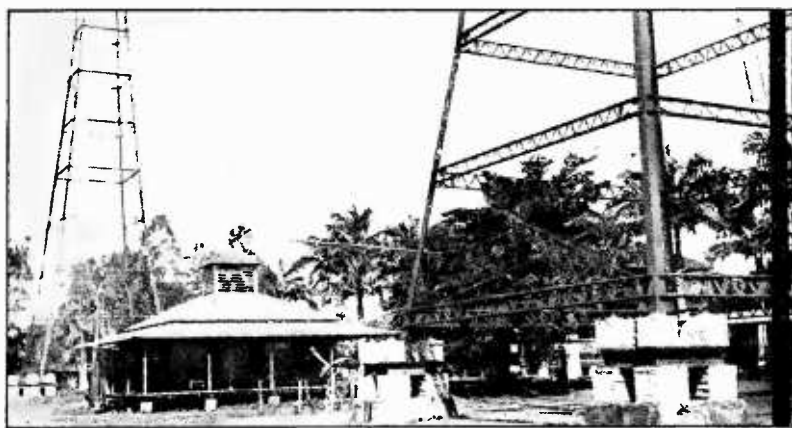
RADIO STATION AT PORT LIMON Headquarters of the United Fruit Company's Costa Rican Division
