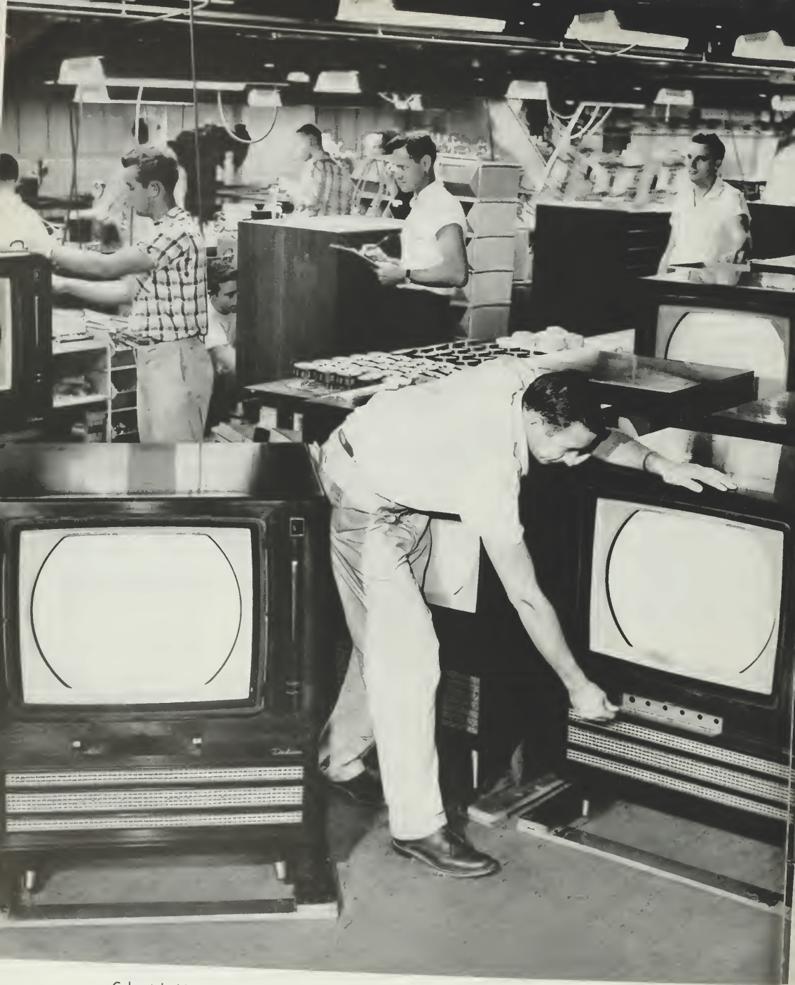
Color television sets in production at the RCA Victor plant in Bloomington, Indiana.
