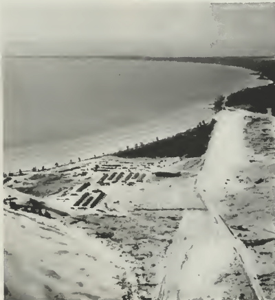
8. Each of the down-range stations, like Eleuthera here, is a technical outpost manned by an average of 80 technicians.
