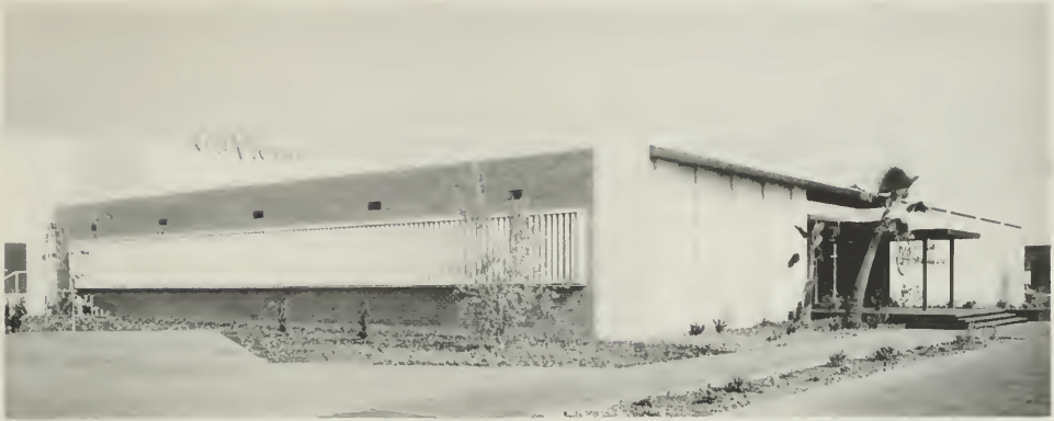
This ultra-modern RCA distribution center in Los Angeles is largest facility of its kind in California.
