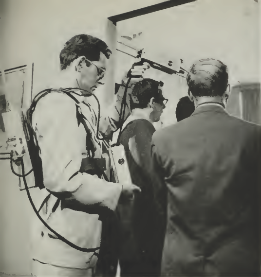
The new RCA transistorized TV camera-transmitter unit features detachable electronic view-finder which enables cameraman to hold camera above eye level and still see the picture he is getting.
