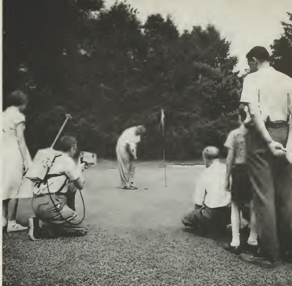
With transmitting range of more than a mile, the portable unit can pick up and send TV signals to base station for network broadcast to provide coverage of outdoor events as shown in this picture.
