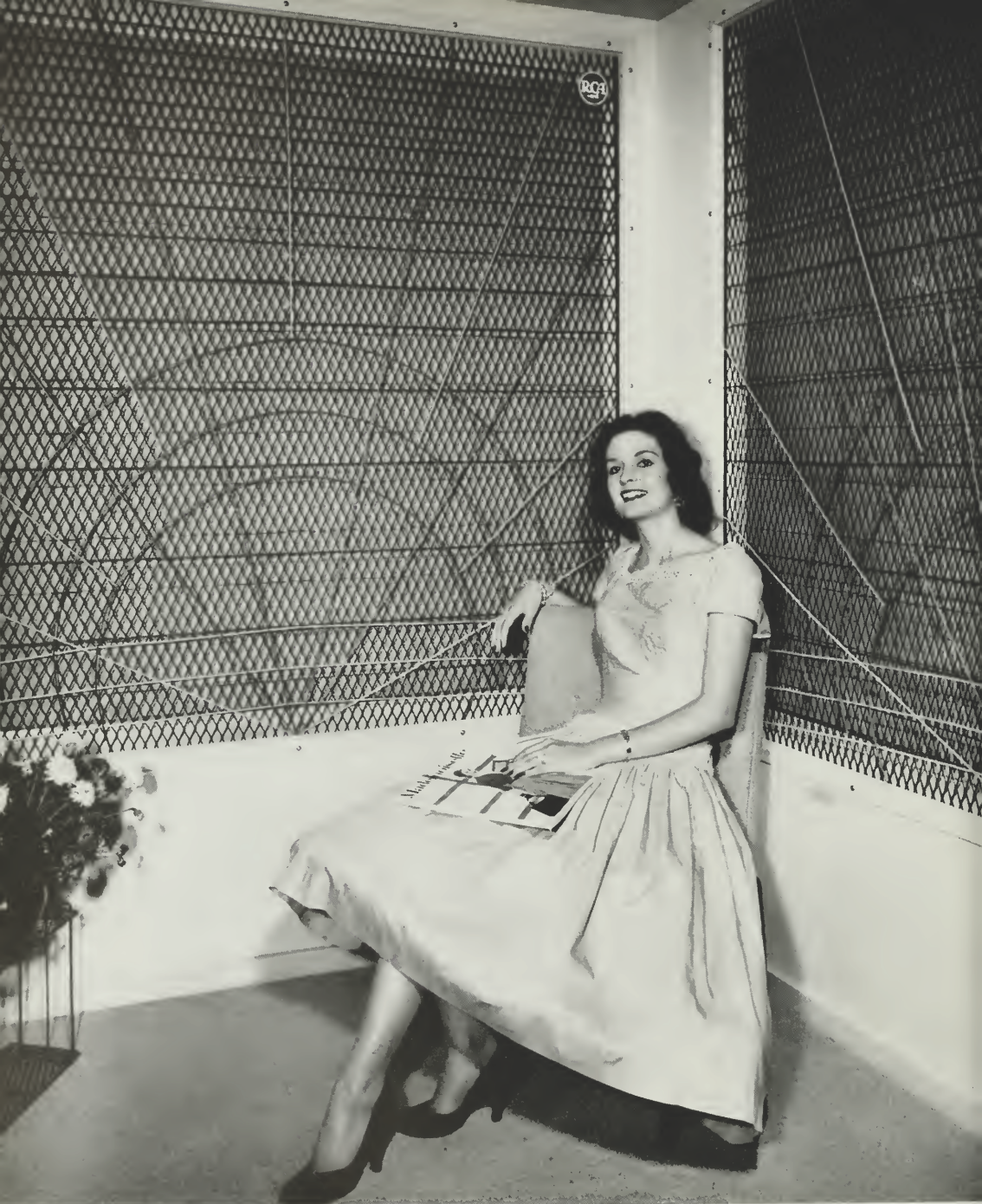
Inside the world's first electronically air conditioned room, at RCA's David Sarnoff Research Center. Cooling or heating are provided noiselessly by wall panels behind decorative grills shown here.
