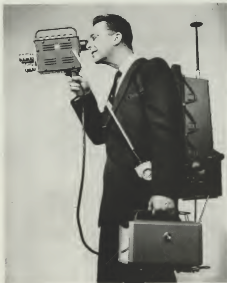
NBC commentator Chet Huntley demonstrates what the well-equipped TV reporter will wear at the conventions. He carries portable TV camera and back-pack transmitter, two-way transceiver for radio communication (in his pocket) and light portable TV set.
