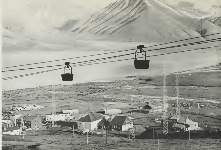
On Spitsbergen, Norwegian island north of the Arctic Circle, this RCA transmitter operates regularly not far from the North Pole.
