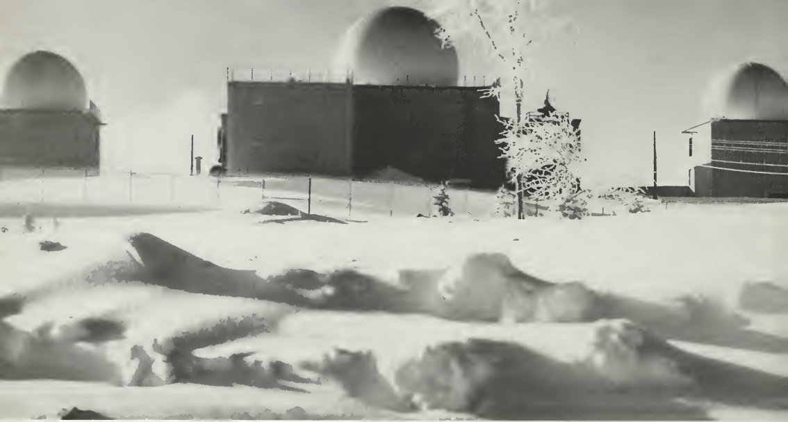
Domes housing electronic equipment stand against winter sky at an RCAF radar station.
