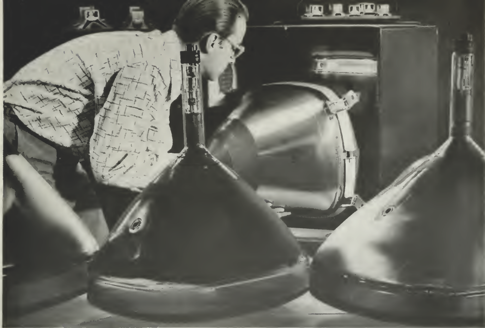
Adjusting a new picture tube for an RCA television set — one of the 5 million produced by RCA.
