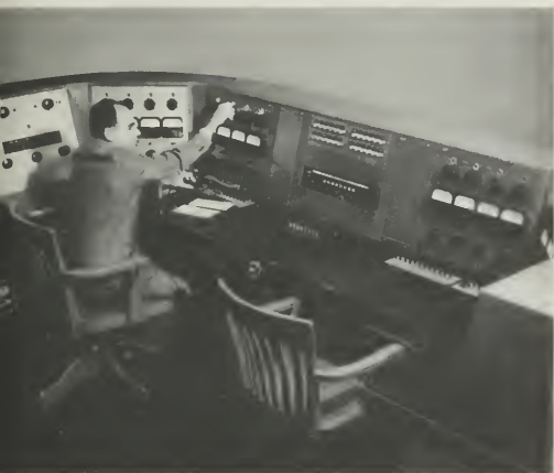
key point in world-wide broadcast service is this control console at RCA Communications in New York.
