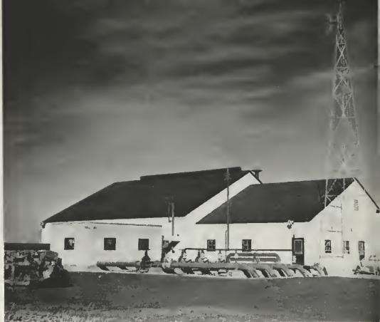
This microwave station at Edmonton, operated by Northwestern Utilities, serves as communications center for 40 mobile vehicles.
