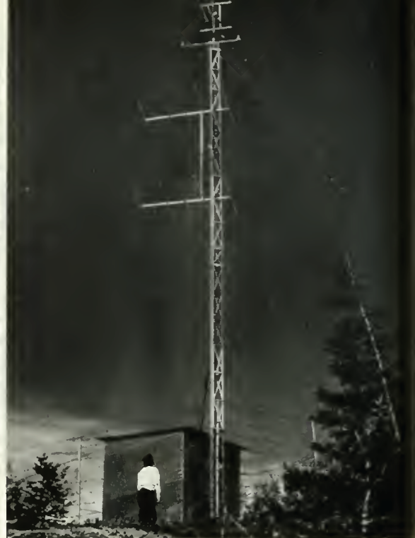
Coaxial transmission lines lead from central television receiving antenna on Mt. Belknap to Laconia, six miles away. At right: Close-up of Antenaplex tower on 2,400-foot mountain.
