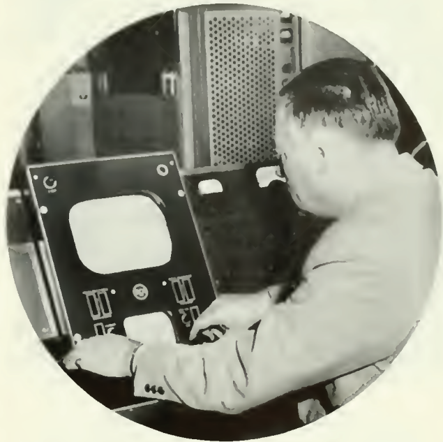
Test pattern shows up on RCA Victor control console installed at CBFT transmitter.
