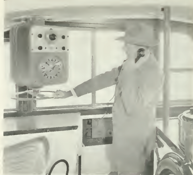
Radiomarine direction finder installed in the wheel-house of the yacht Seaquester .
