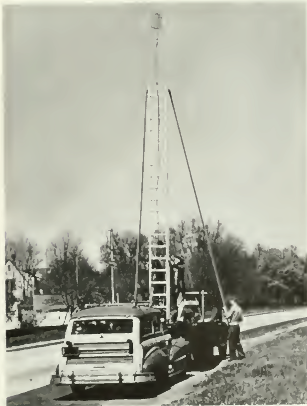
Television engineers raise a portable antenna to check the strength of UHF signals transmitted by the RCA-NBC station at Bridgeport, Conn.
