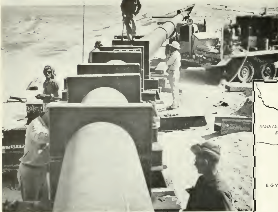
Left: Section of Tapline conduit which carries daily flow of 300,000 barrels of oil over 1,000 mile route shown below.
