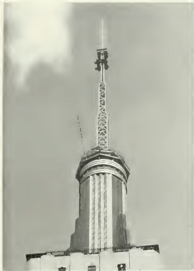
Station WNBT recently began regular transmissions from the new 215-foot television mast atop the Empire State Building.
