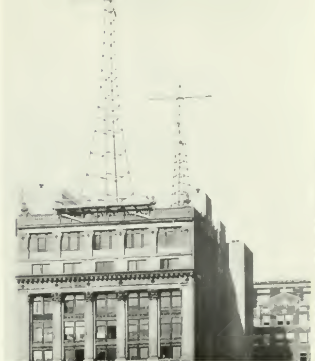
Dual antennas for stations WJZ-WJY were erected on the roof of Aeolian Hall in New York City.
